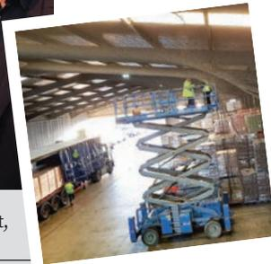
The team installed sparrow netting using a framework of steel wire fixings, strainers, clips and guide brackets to hold approximately 2,400 square metres of netting.
